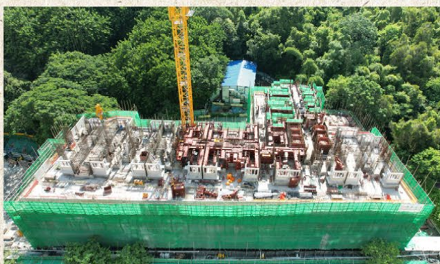
Public housing development at Hin Fat Lane, Tuen Mun, N.T.
